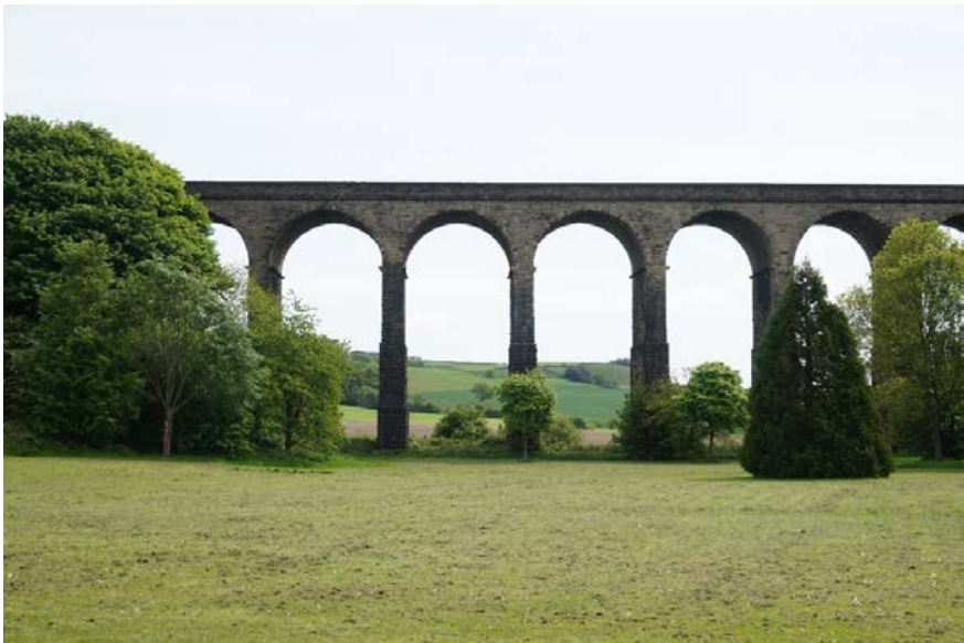
5 Across Water Hall Park to Viaduct
